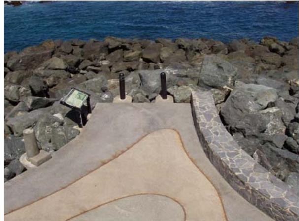
**Figure 5-7 Close-up of Existing Stone Seat Wall and Bollards at the “Water Battery”**
