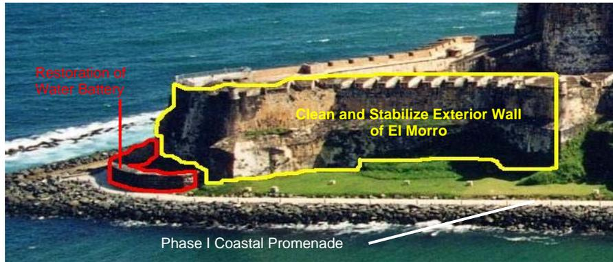
**Figure 5-5 Phase I Coastal Promenade, Water Battery, and Wall Area Proposed for Improvement**
