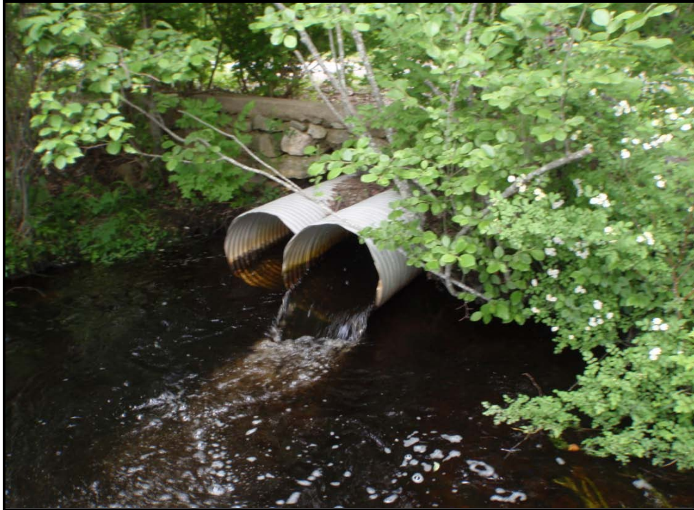
Figure 6. Teal Drive culverts, Factory Brook, South Kingstown, RI, 2011. The culvert perched on the right is higher than the culvert on the left and both culverts provide poor fish passage with varying stream flows.
