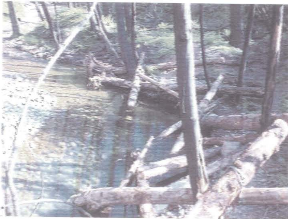
Figure 29: Completed placement of woody debris in stream
