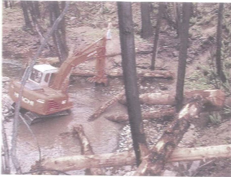
Figure 28: Heavy Equipment Working in Stream
