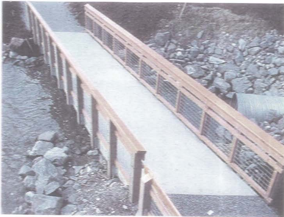
Figure 35: New Fever Creek Bridge
