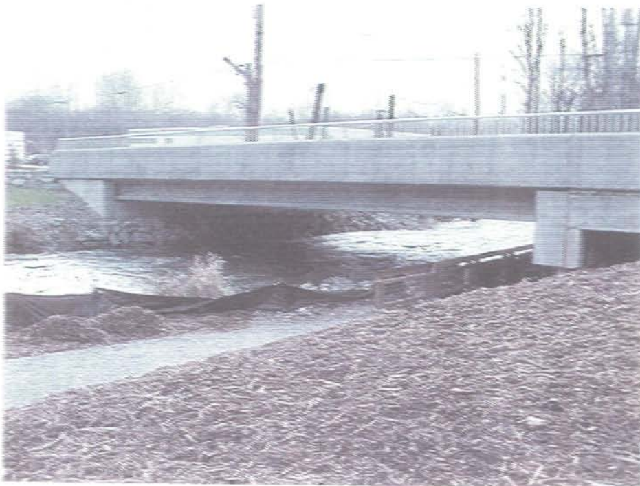
Figure 36: New Valencia Street Bridge
