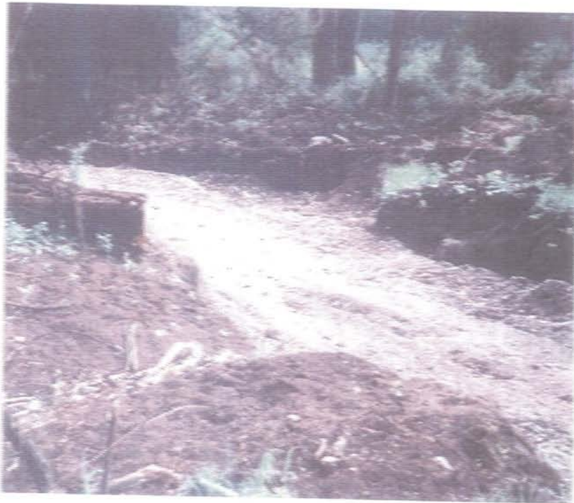
Figure 19: Hanna Creek Remediation (Before)
