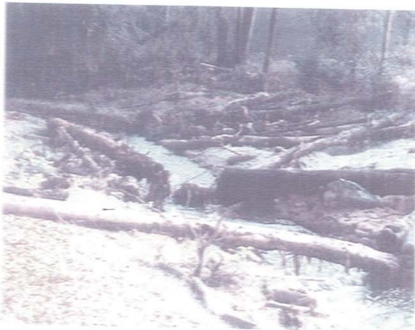
Figure 20: Hanna Creek Remediation (After)
