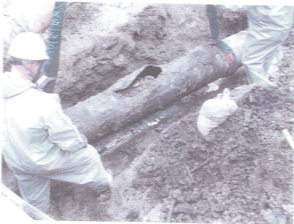
Figure 3: Excavation of Pipe
