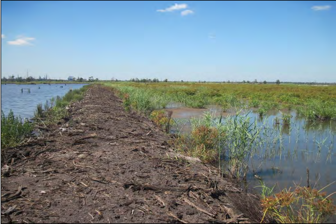
Photograph 33 – A representative view showing the berm separating the easement from the sand filled cells. Tidal water has begun to erode the berm. This photograph was taken facing west at 30.078089, -94.023803.
