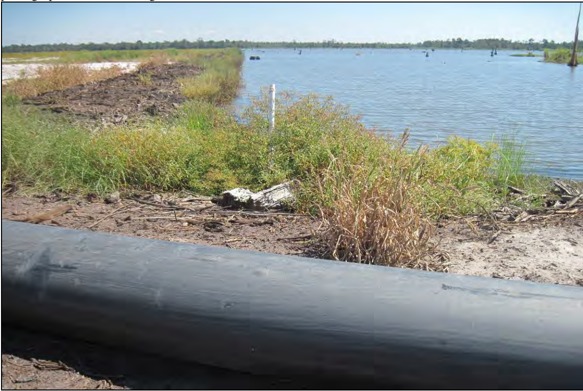
Photograph 18 – A view showing the pipeline corridor that is being constructed along the northern boundary of the subject property. The trench has been dug and the spoil pile has been built up above the high tide water level. This photograph was taken facing east from the northwest corner of the subject property at 30.07797, -94.029181.
