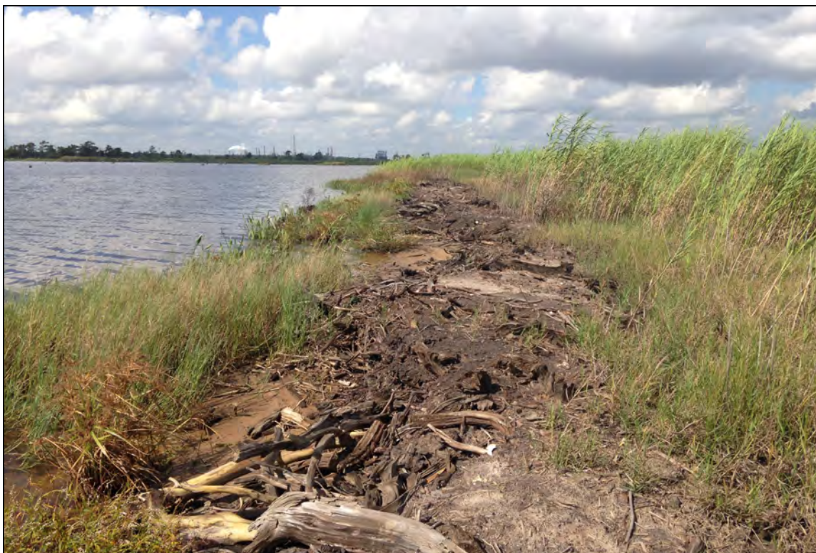
Photograph 3 – Another view west along the levee. Portions of the levee are in poor condition due to the quality of materials that were used in constructing the levee.
