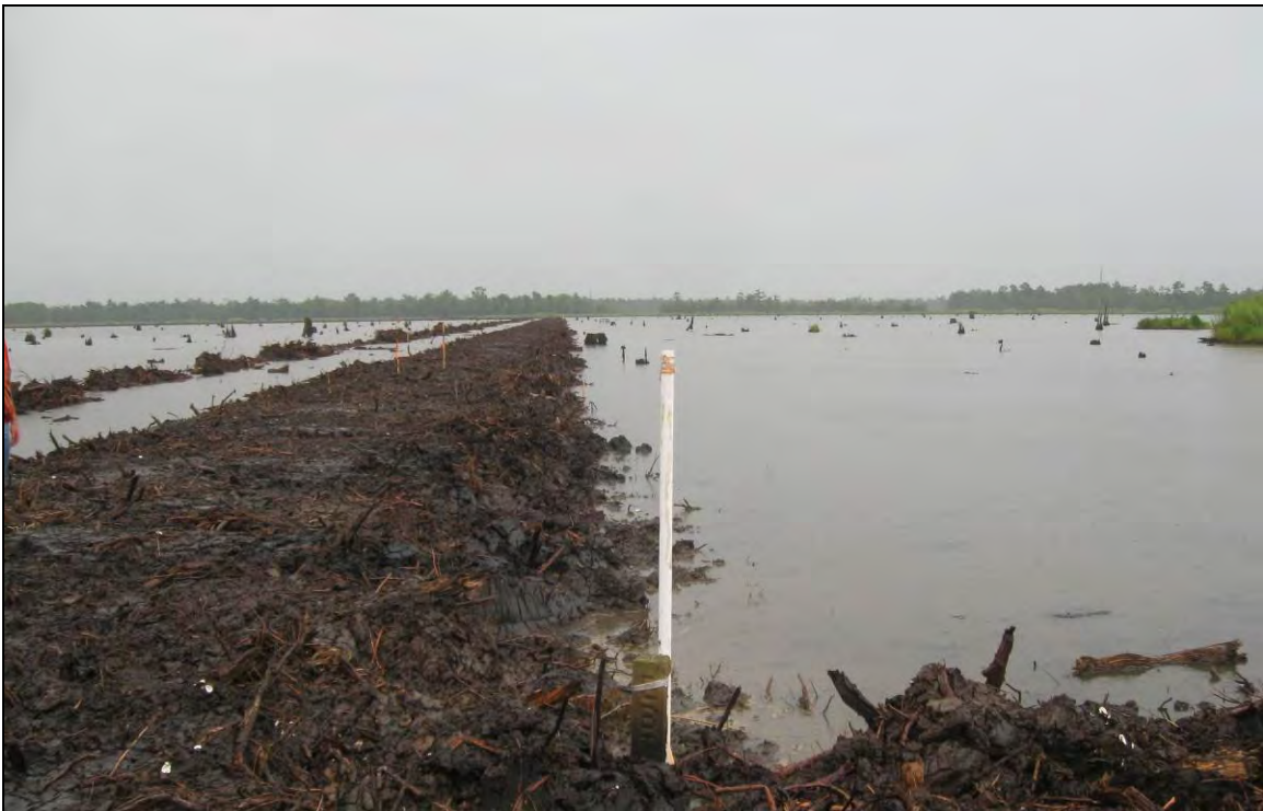
Photograph 18 – A view showing the pipeline corridor that is being constructed along the northern boundary of the subject property. The trench has been dug and the spoil pile has been built up above the high tide water level. This photograph was taken facing east from the northwest corner of the subject property at 30.07797, -94.029181.
