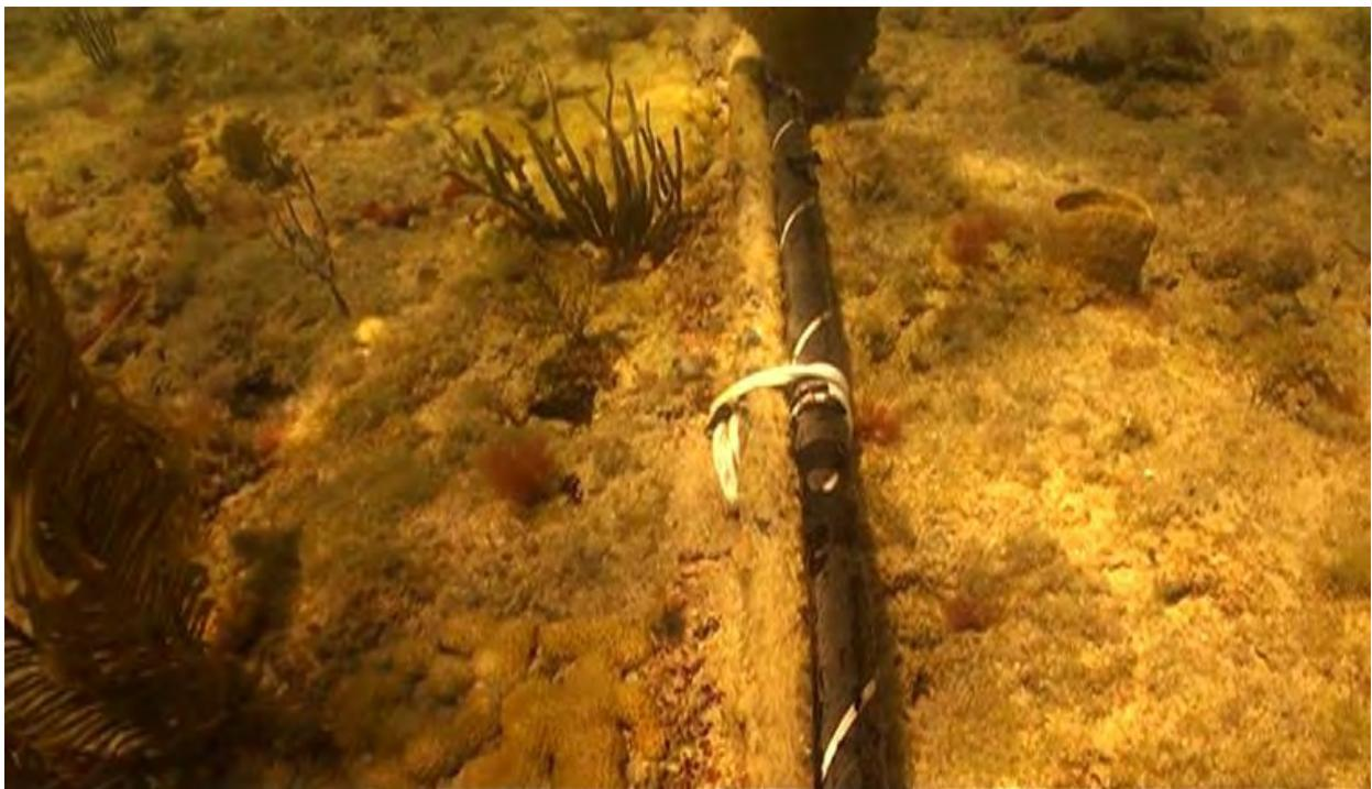
**Figure 3: Gateway and SCMS cables on seafloor (bundled with previously laid cable)**
