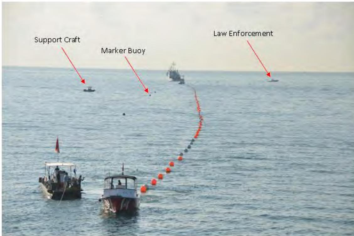
Figure 2: Preparing to attach SCMS cable to shore ending lead in line
