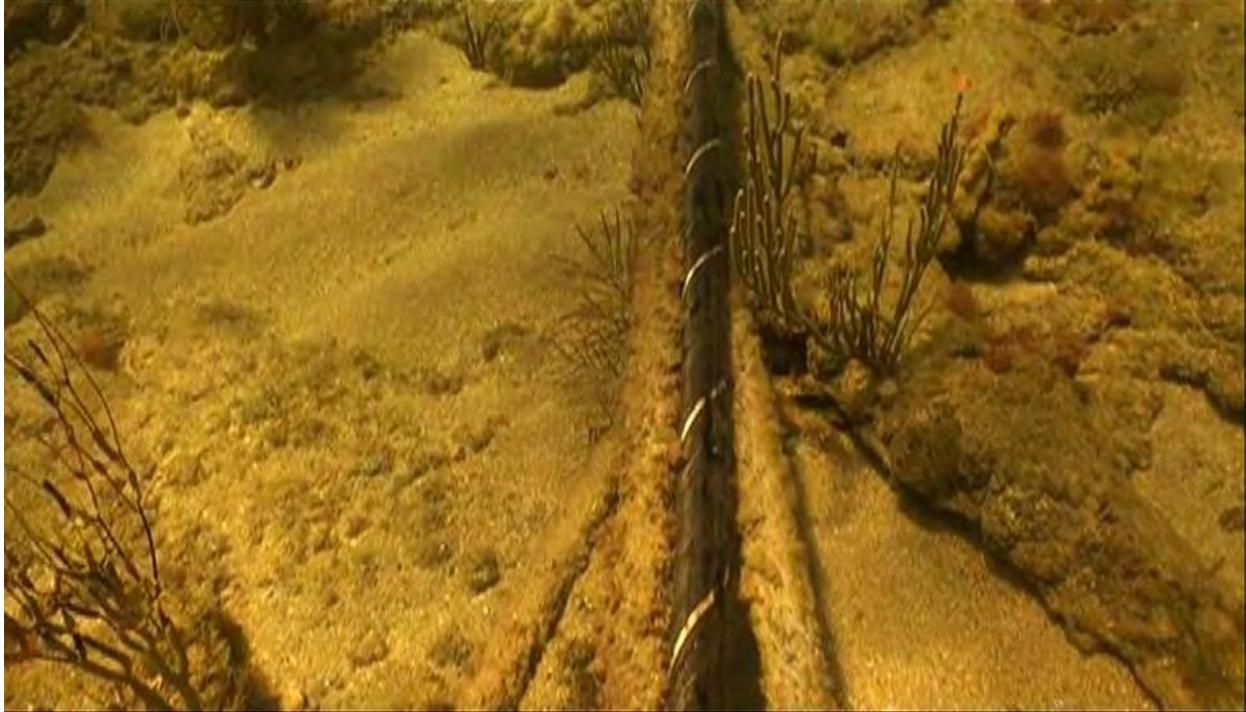
**Figure 4: Gateway and SCMS cables on seafloor joining other cables heading to the beach**
