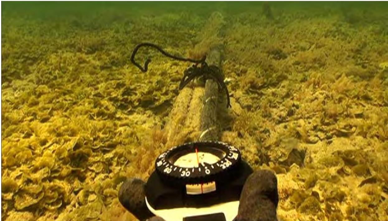
**Figure 5: Gateway, SCMS and other cables secured to seafloor at hard point**
