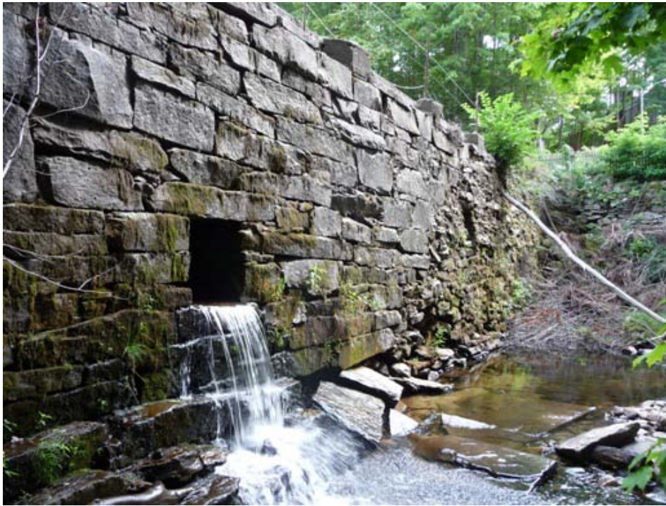
Figure 4. Downstream face of the Bartlett Rod Shop Company dam with mid-level outlet, releasing Amethyst Brook flows.
