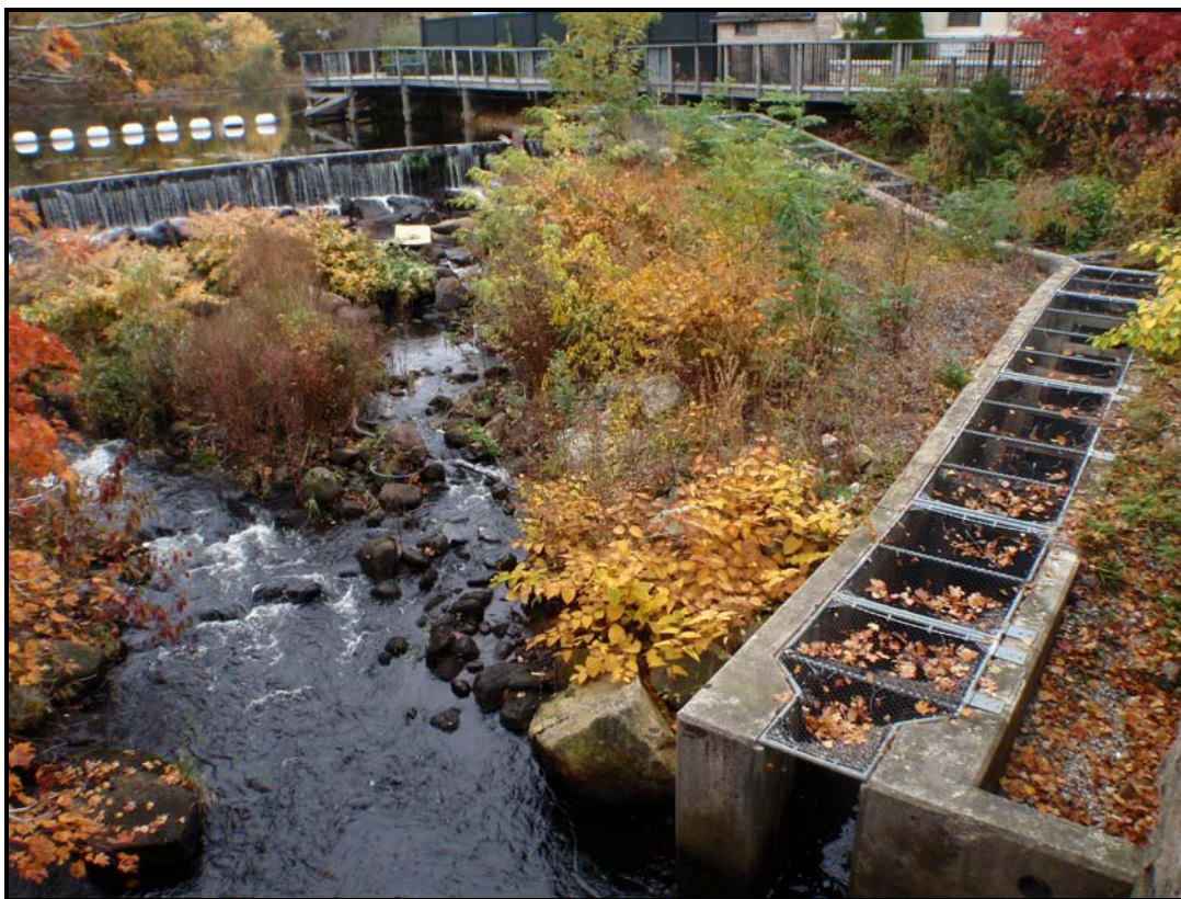
Figure 2. Main Street dam and existing fishway, 2011, Wakefield, RI
